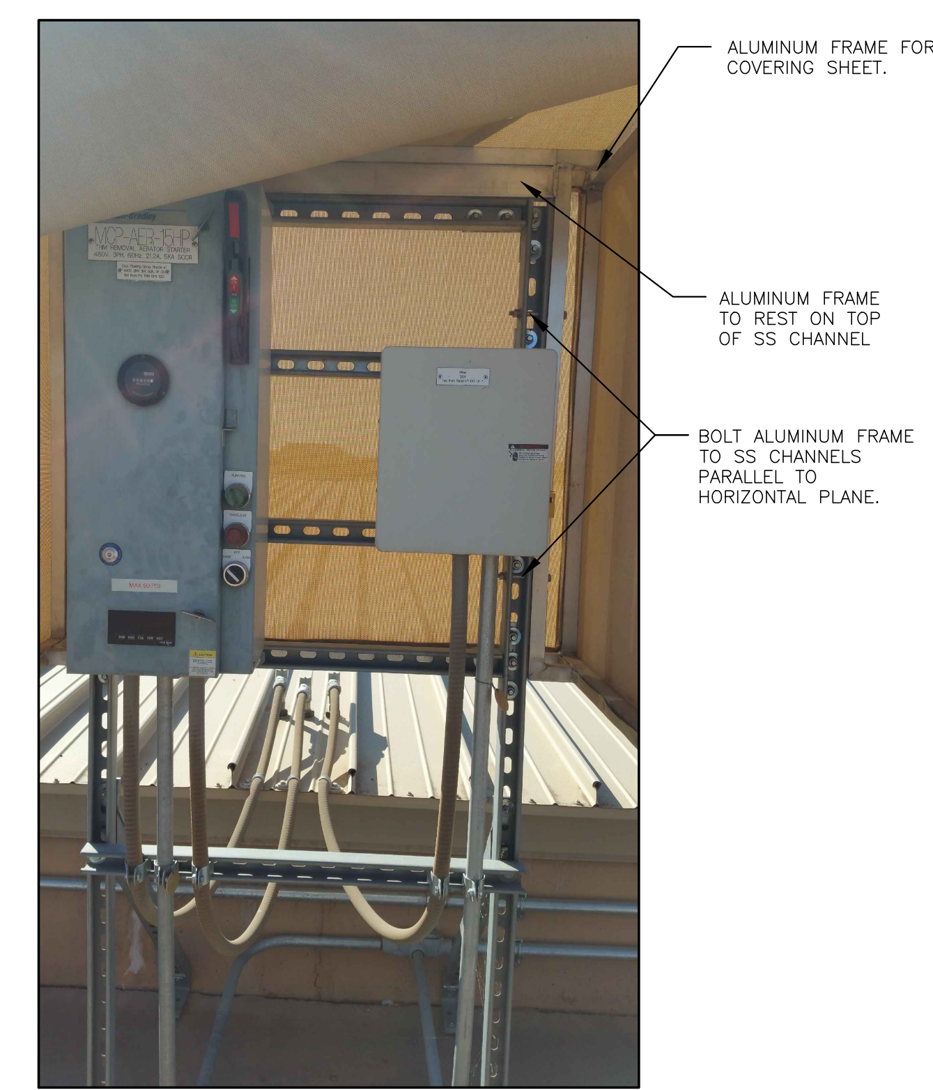
FABRIC COVERED SUNSHADE DETAIL AAA NOT TO SCALE
